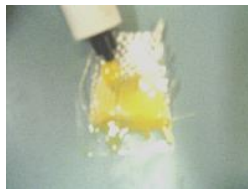
2. Apply resin to tab/mesh until fully moist.
